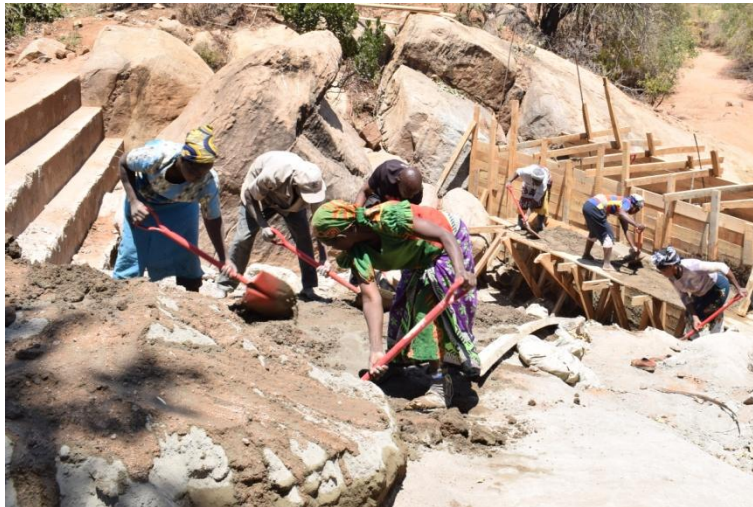
Above top: Kinuvu SHG mixing cement for their sand dam Bottom: Wendo wa Matoki SHG mixing cement for their sand dam
