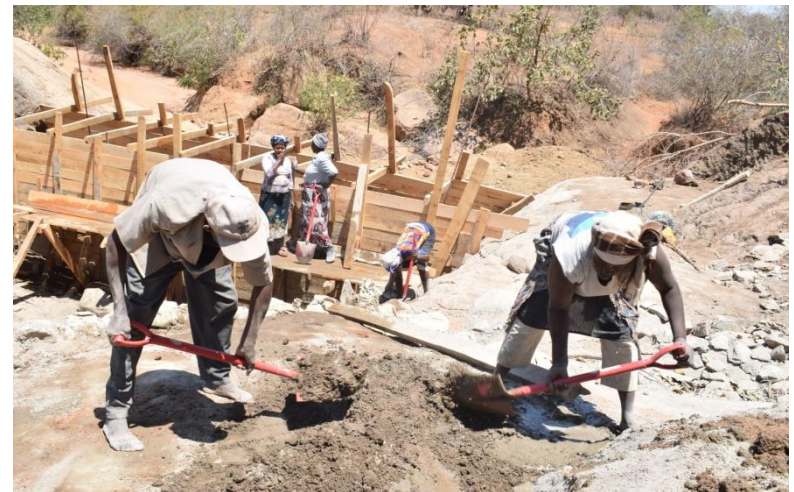
Wendo wa Matoki SHG excavating bedrock (above) and mixing cement (below) in preparation for their sand dam
