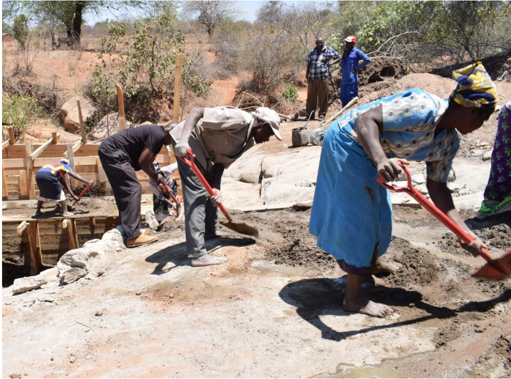
Above: Members of Wendo wa Matoki mixing cement for their sand dam
