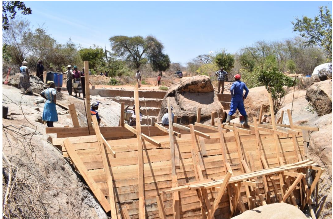
Above: Timber shuttering provides the framework for Wendo wa Matoki SHG's sand dam
