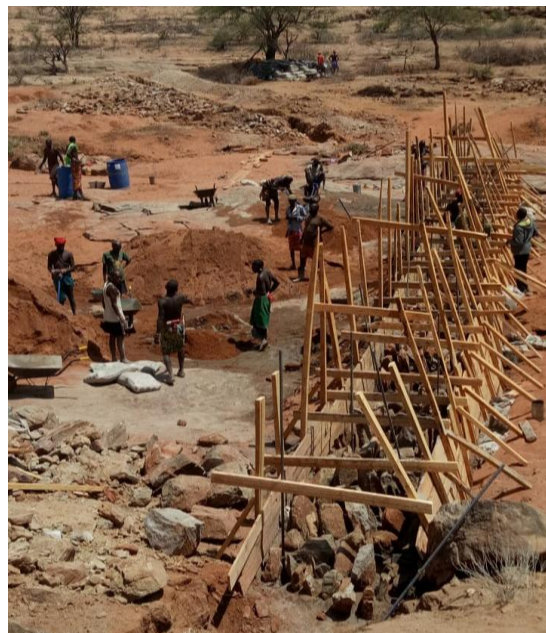
Tassia E (Lekurruki) and Mokori (Oldonyiro) sand dams under construction
