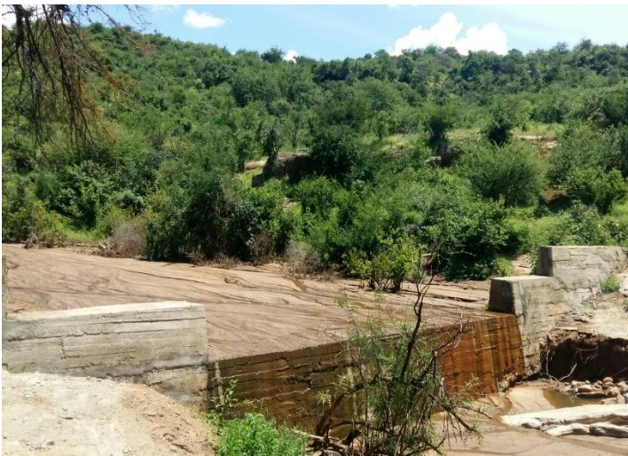
Nolasuri (top left), Junction (top right) and Tassia B (bottom left) completed sand dams in Lekurruki Conservancy, and Kitagezi (bottom right) completed sand dam in Oldonyiro Conservancy
