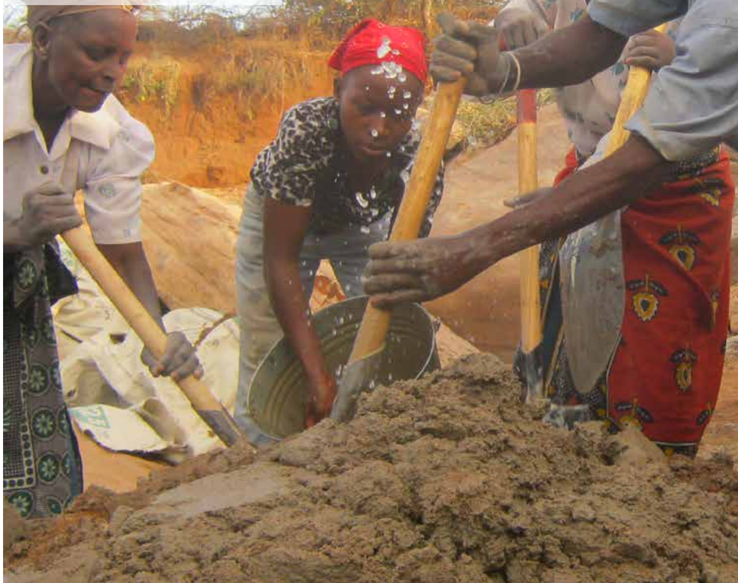
Photo: Members of the Stay ya Thange self-help group, southeast Kenya, mixing cement for their sand dam.
