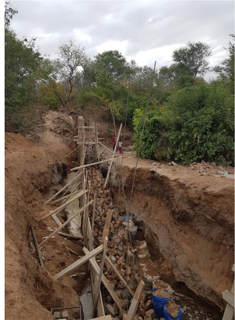
Doca sand dam under construction
