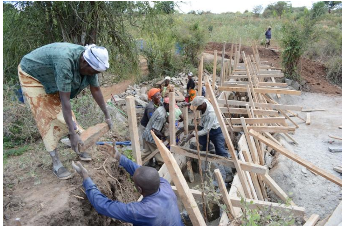
Above top: Tukile SHG at the trench dug for the wing walls of their dam
