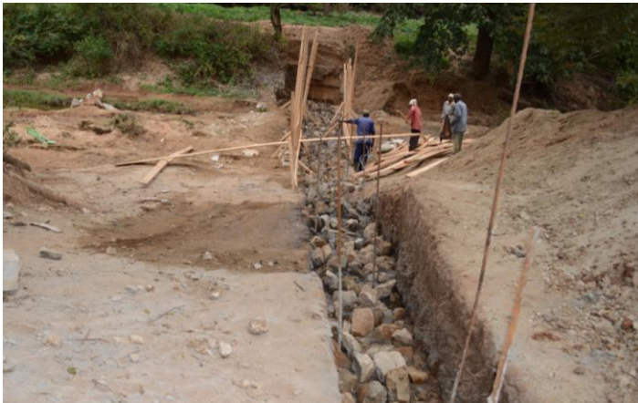
Above top: Tukile SHG at the trench dug for the wing walls of their dam
