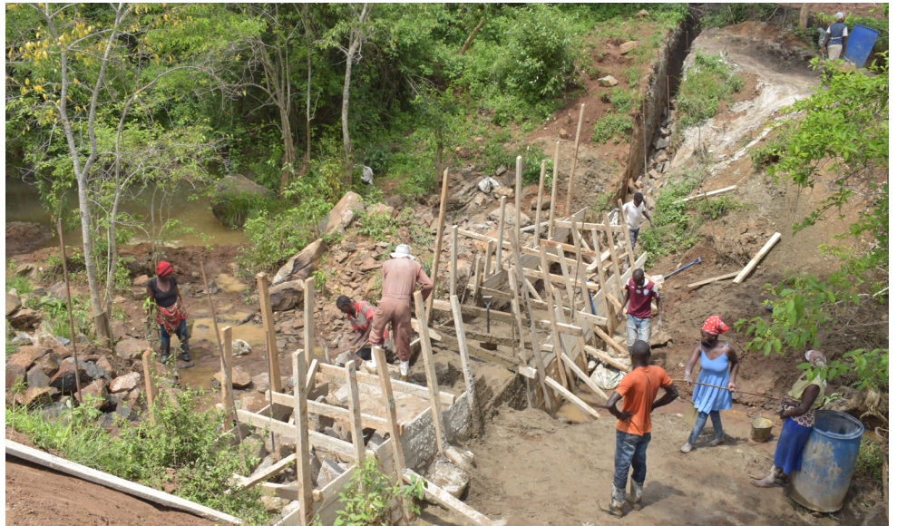
Tyaa Tito’s sand dam, mid-construction, December 2020
