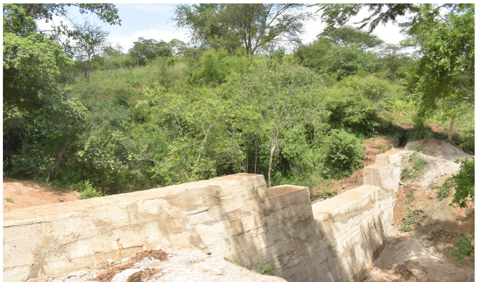
The self-help group’s completed sand dam, January 2021
