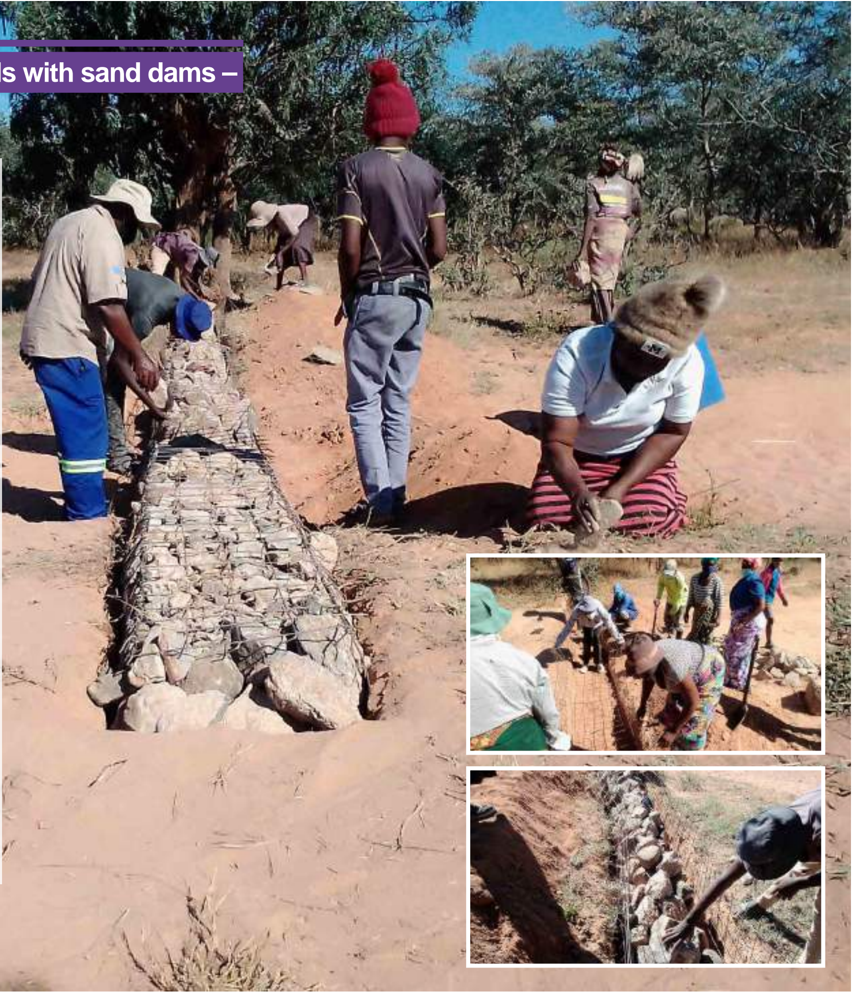
Photos: Stages of stone gabion construction near Nkumbu, Zimbabwe. First there is the digging of the trench and setting out of the wire casing, which is then filled with locally collected stones, before everything is secured with the wrapping of wire.
